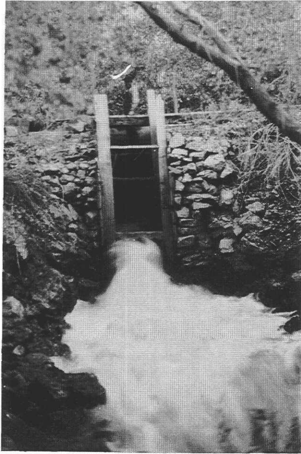
Figure 24. Canal sluice (courtesy Fern Reeve).
